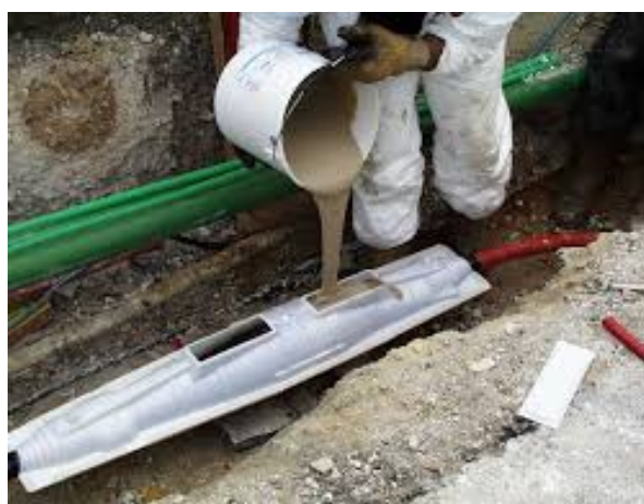
Fig. 2 Compound filling process in joint kit
